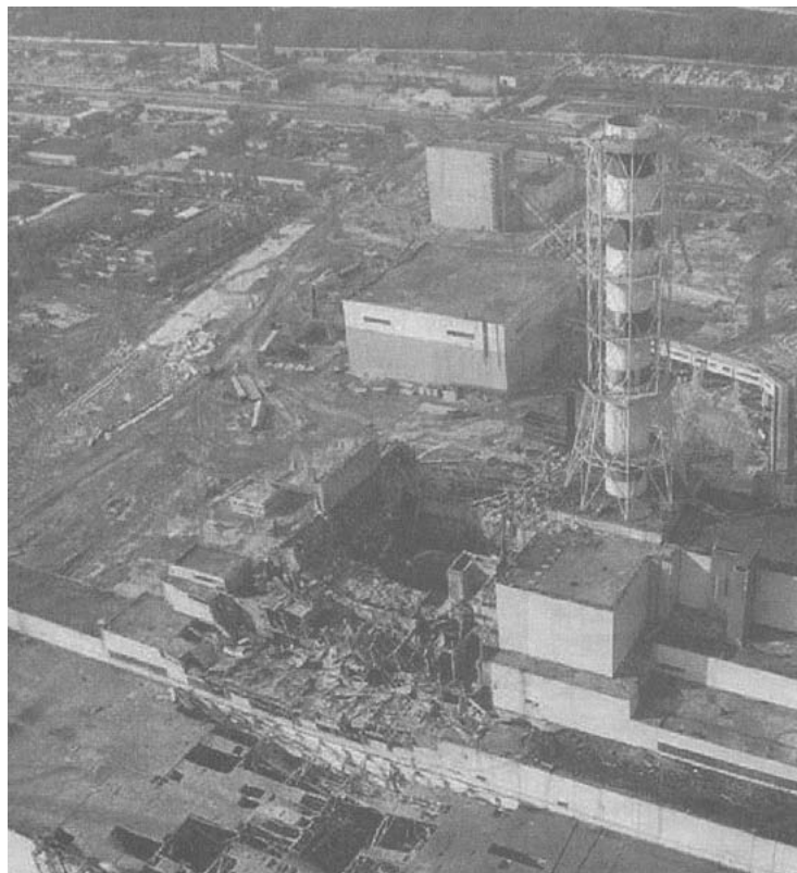
Figure 12.3. The destroyed reactor at Chernobyl. Unlike U.S. reactors, this one had no concrete containment building.
