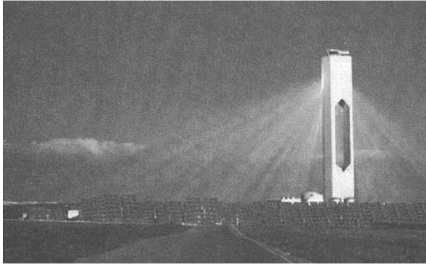
Figure 6.1. Solar power plant near Seville, Spain. The mirrors focus sunlight onto a boiler, and the resulting steam runs a turbine that produces electricity.
